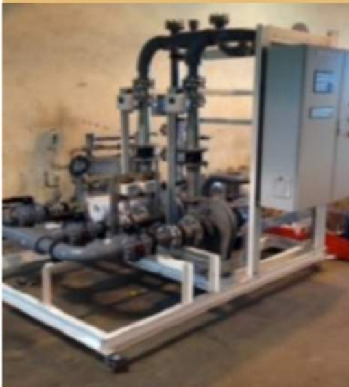
Ventilation Skid for Trawsfynydd
